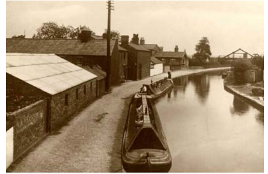
View of the Canal-side buildings taken from Brooks Lane Bridge. In the middle ground is the Canal terraced housing, mainly lived in by boat families. Beyond that is the storage building and the Canal Inspectors office. Allan Earl
