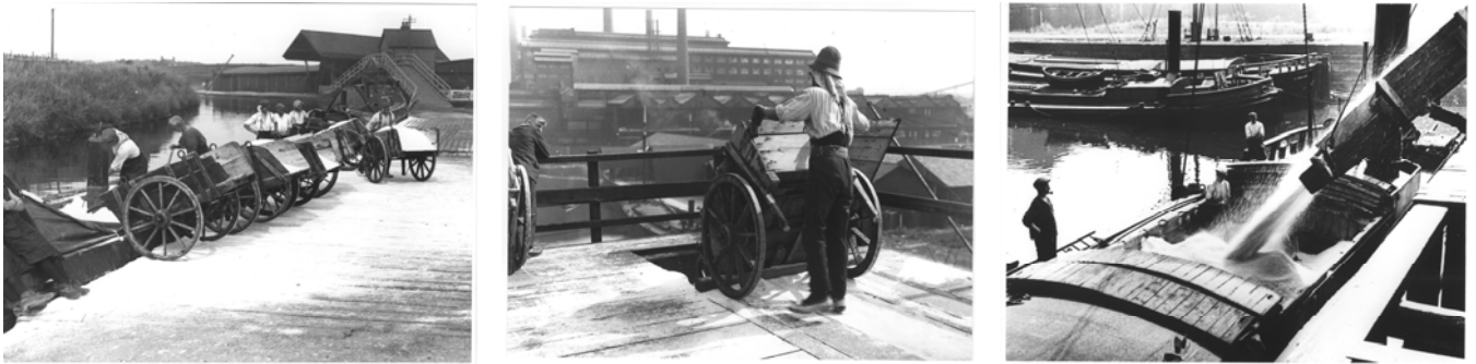
Digging out the common salt and loading into barrows at the transfer point, the chutes were placed over the boats. Anderton Boat Lift. Photos supplied by The Waterways Trust, Ellesmere Port ©
